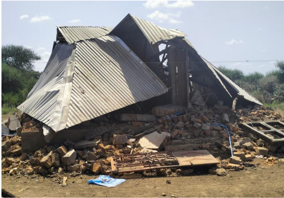
Home demolished by state forces on 8 May 2024. Families are now sleeping outside.
